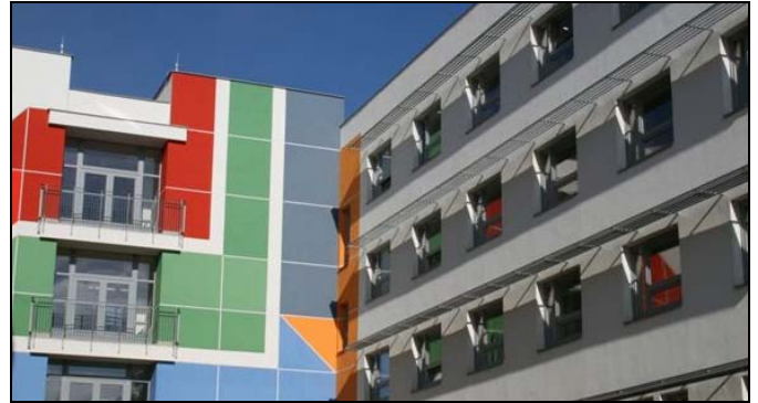
The new FDR High School building in Brno opened November 16.
